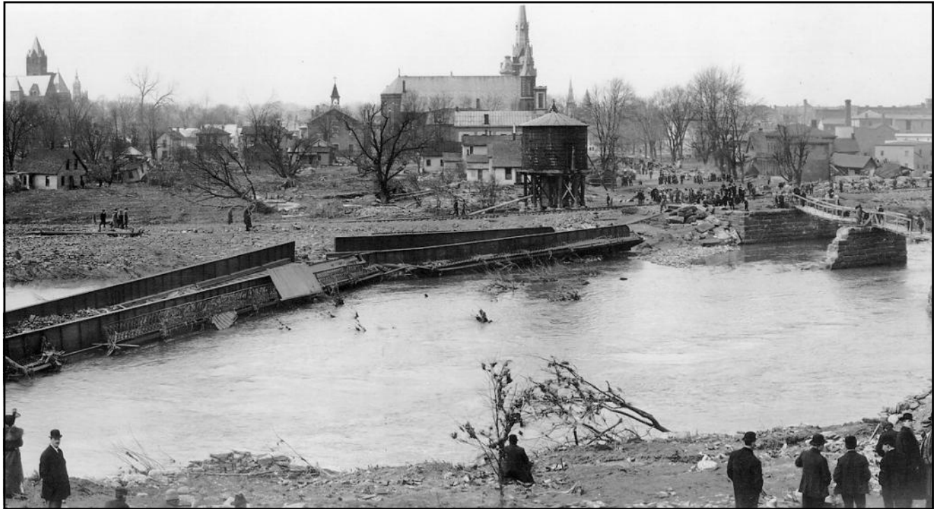
Looking west across the Olentangy River at William Street after the Flood of 1913
