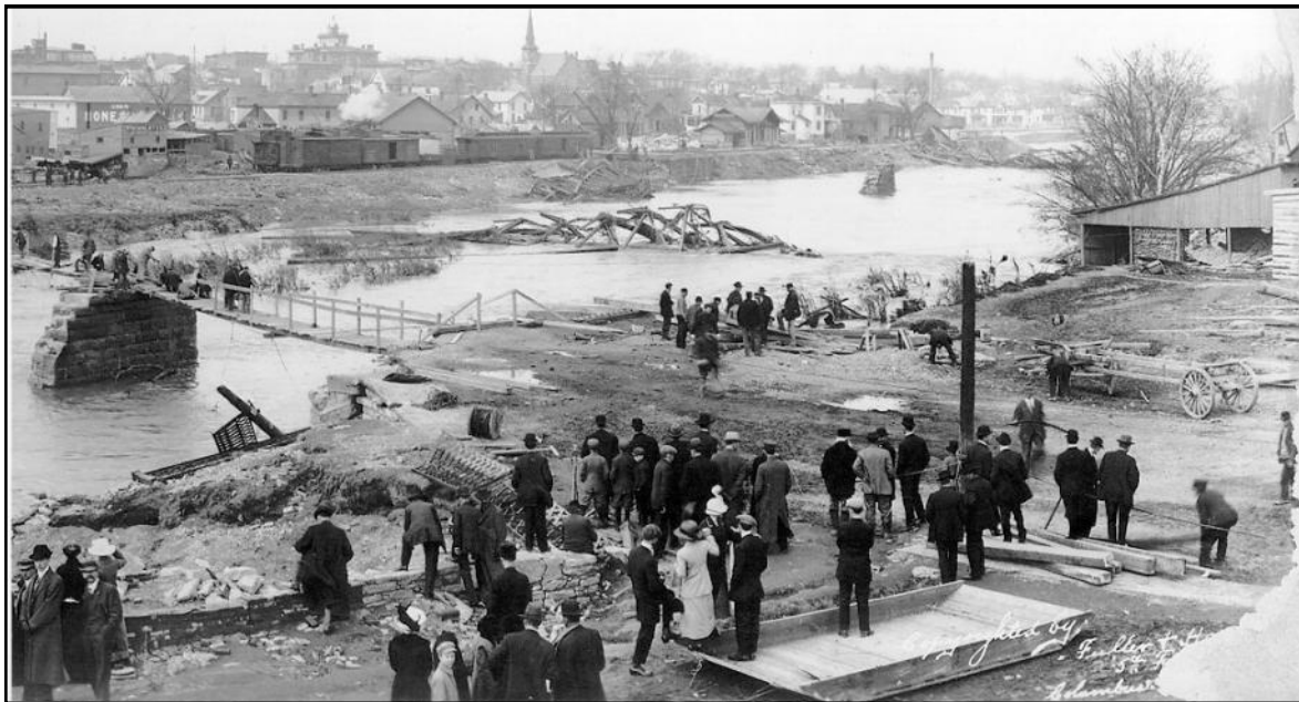
Temporary bridge across the Olentangy River at William Street after the Flood
