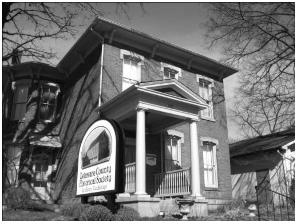
The newly repainted Nash House
