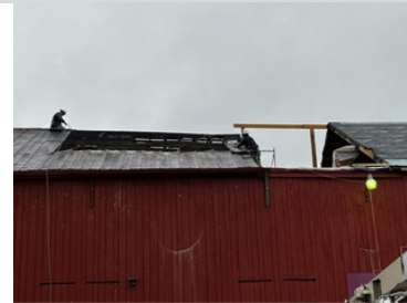
In January, removal of the south side began.
