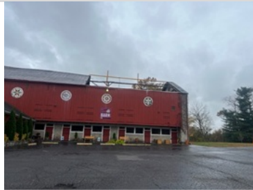
The north half of the roof was removed first.
