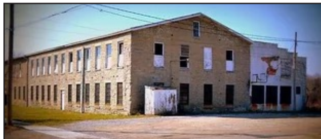
This photo is of the abandoned Flax Mill and Warehouse, located on Flax Street. The building later housed the Delaware Chair Factory.
